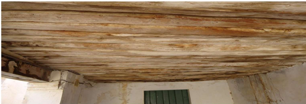
Figure 5. Wood roofs khenguet Sidi Nadji Source: Own elaboration (2023)
